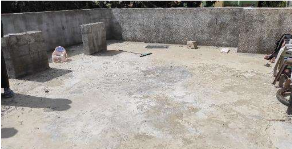
Proposed site for PV installations at HH2
