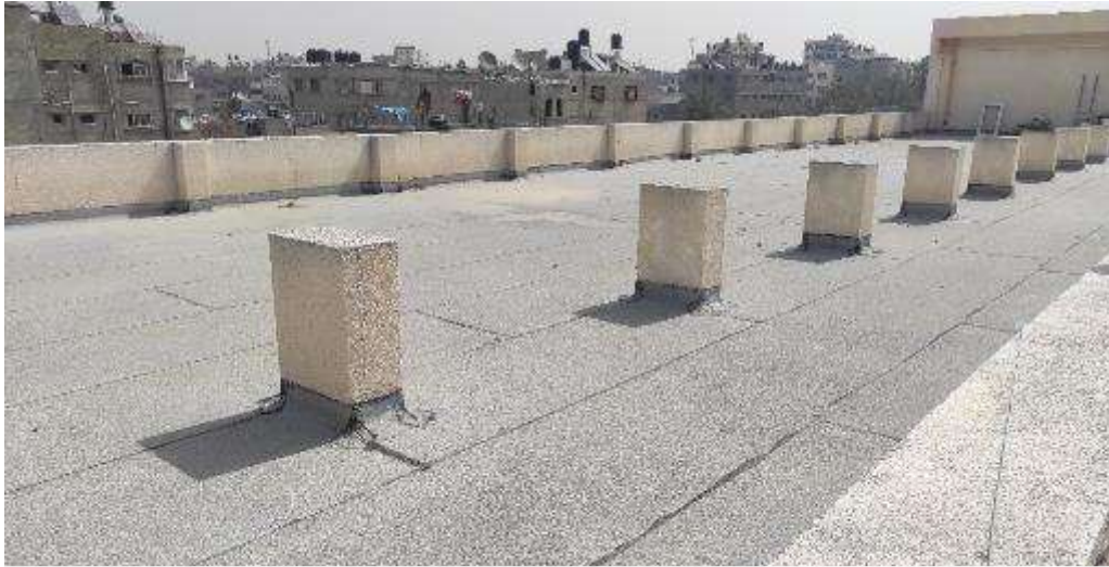
Proposed site for PV installations at Sumaya Bint Kheyat School
