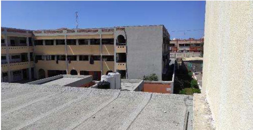
Western border of the proposed site for PV installations at Hatem Atta'i School
