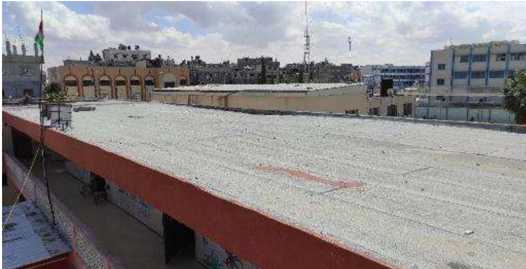
Proposed site for PV installations at Hatem Atta'i School
