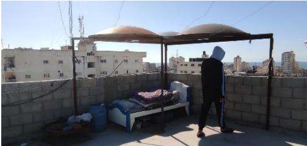
Proposed site for PV installations at HH5 (The bed and the steel cover will be removed to create enough shade-free area for the installation of the system)
