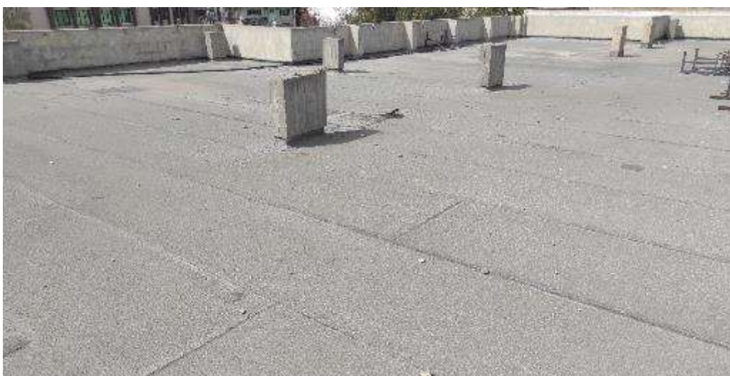
Proposed site for PV installations at Al Rafi'i School
