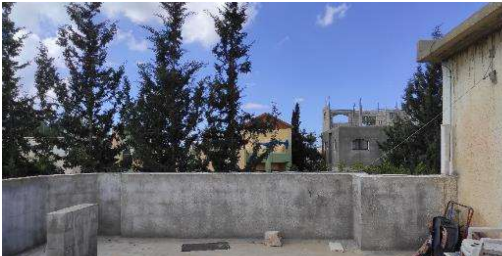
Western border of the proposed site for PV installations at HH2
