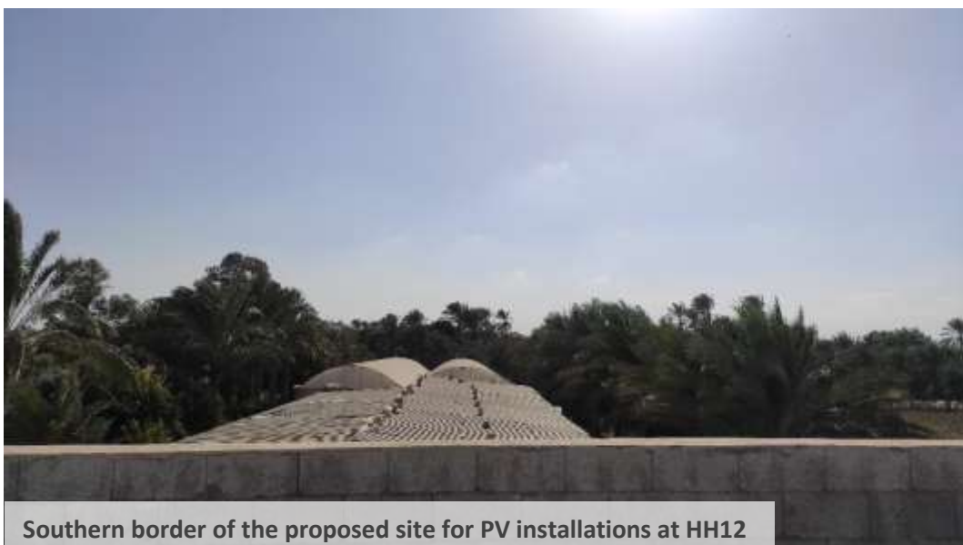
Proposed site for PV installations at HH12
