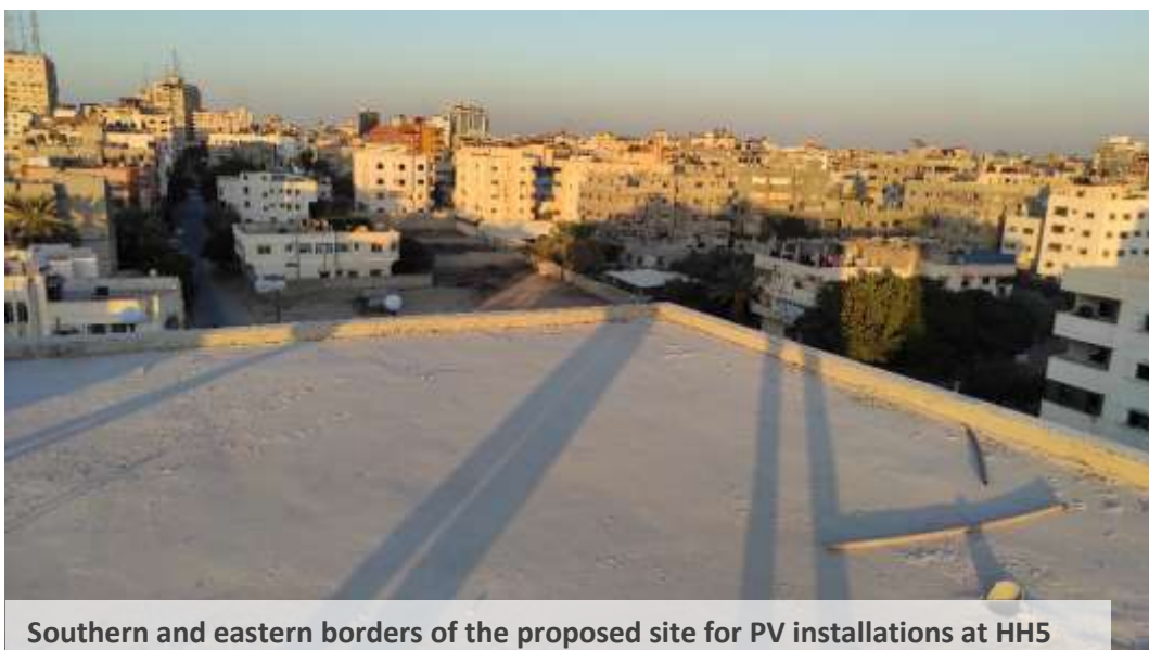
Proposed site for PV installations at HH5 and its southern border
